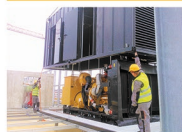
DACH BUDYNKU CREDIT SWISS
